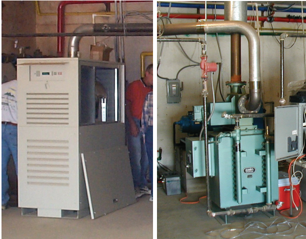
The Capstone Model 330 microturbine combined with heat recovery system installed at Colorado Pork.
