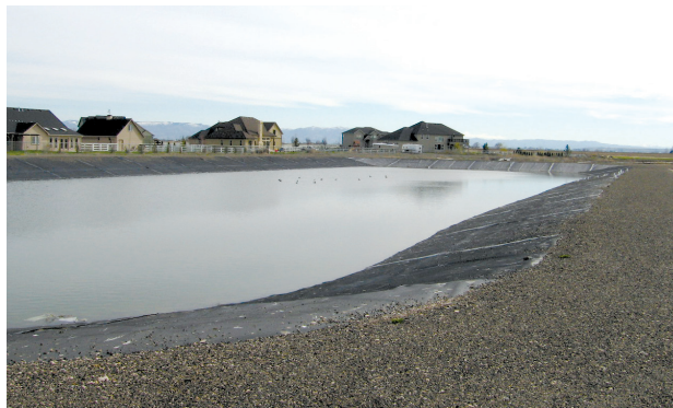
The 50-home Trellis Subdivision in Eagle, Idaho, that uses the International Wastewater Systems, Inc. Model 6000 SBR.
