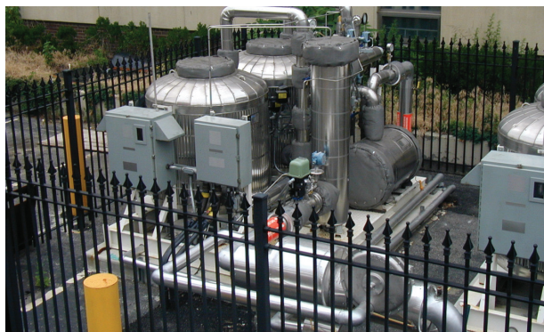
The USFilter/Westates Carbon gas processing unit installed at Red Hook Water Pollution Control Plant.
