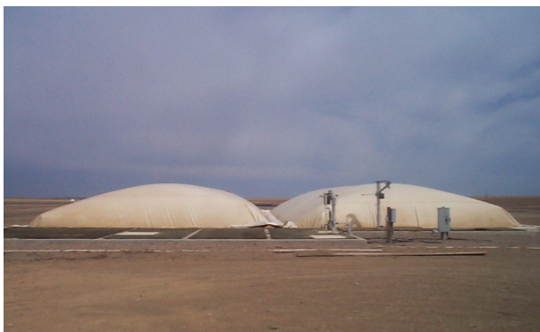
The anaerobic digester at Colorado Pork in Lamar, Colorado.
