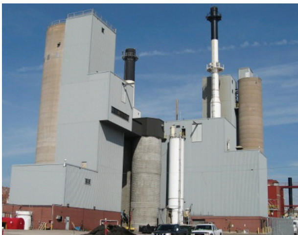
The University of Iowa main power plant.
