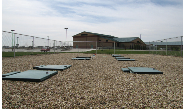
A view of the Model 6000 SBR following installation at the Trellis Subdivision in Eagle, Idaho.
