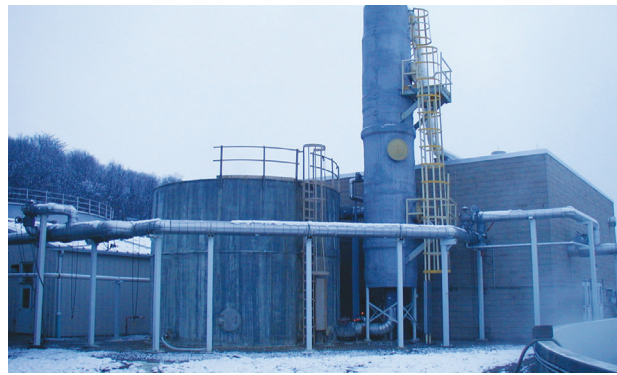
NATCO THIOPAQ ® system with aerobic bioreactor and scrubber installed at a water pollution control facility.
