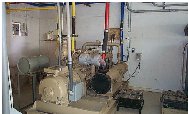
The Martin Machinery Caterpillar Model 3306 internal combustion engine combined heat and power system installed at Colorado Pork in Lamar, Colorado.
