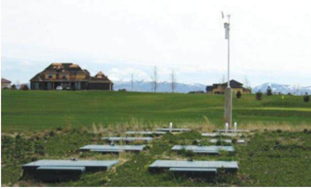
A finished view of the Model 6000 SBR installation at the Trellis Subdivision in Eagle, Idaho.
